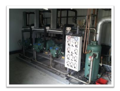
ACE Refrigeration also recently installed a new screw compressor pack for William Sword Bakery as they required R22 Replacement for their Spiral Freezer.
